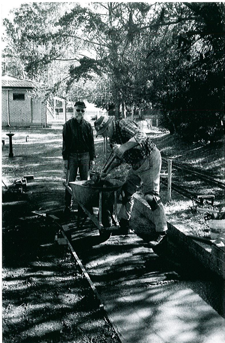
Left. David Thomas delivering the concrete For Lionel.
